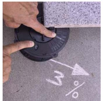
The arrow with the no. 3, shown on the head of the slope corrector, must be positioned in the same direction as the slope which you already marked before (see 2nd step). The head of the pedestal will be water level in each direction. After placing the pedestal under the tile adjust it to the necessary height.
