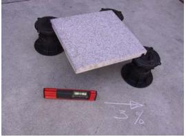
1st step: Place the electronic leveller where the pedestal would stand, to know the value of the slope, as well as the direction of the slope to be corrected.
